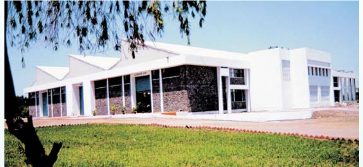
The Ahmednagar factory - manufacturing DC Motors
